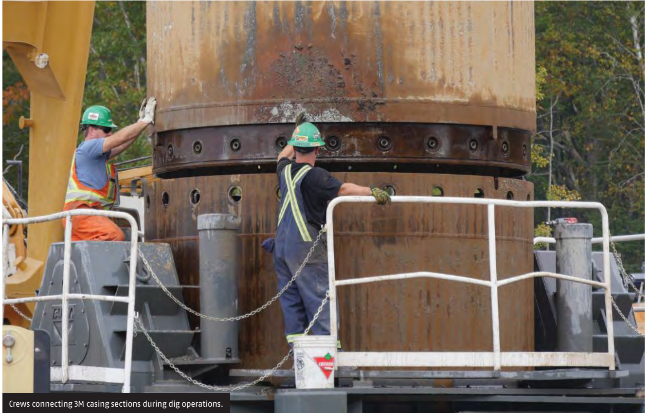
Crews connecting 3M casing sections during dig operations.
